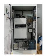
• Irrigation Inverters for the Farming Industry. 12-pulse inverters with step-down input transformers and step-up output transformers to control medium voltage AC motors. Example: 900 HP, 1500 HP. Customer: Priest Electric.
